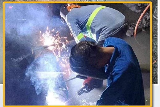
Ongoing repair of the leaking 300mm steel pipe near FSUU Gym as of 3:43 am of June 2, 2024
