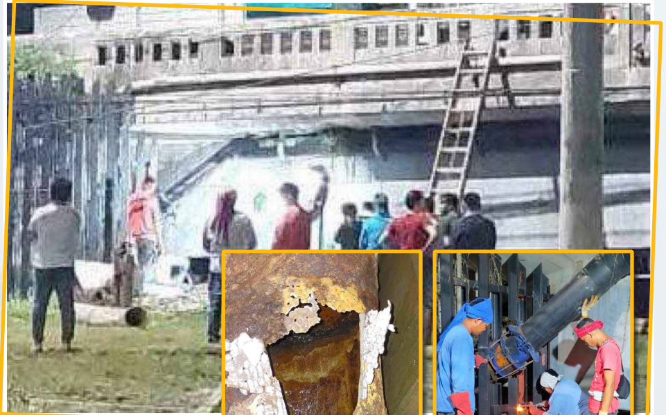
The leak repair of the 250mm steel pipe at Datu Silongan as of 12:15 am of June 2, 2024
