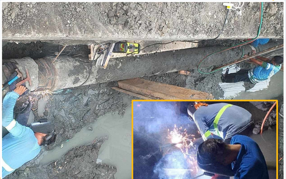
Ongoing repair of the leaking 300mm steel pipe near FSUU Gym as of 3:43 am of June 2, 2024
