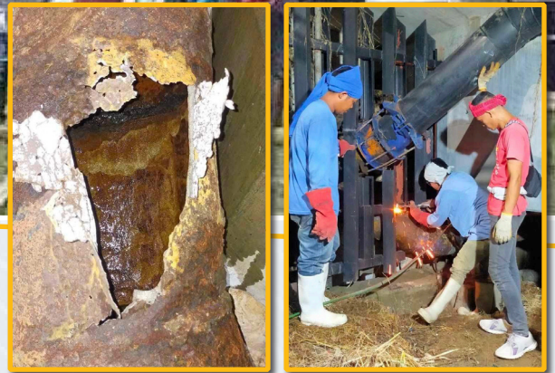
The leak repair of the 250mm steel pipe at Datu Silongan as of 12:15 am of June 2, 2024
